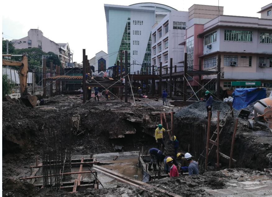
Adventist Medical Center Manila 5 Storey Steel Parking Building
