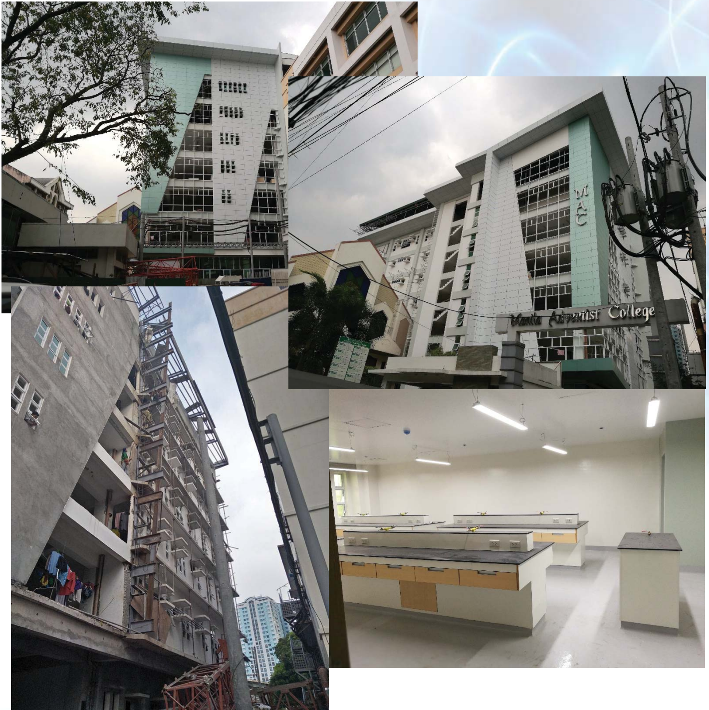
Manila Adventist College 7 Storey School Building with Top Floor Gymnasium & Laboratories
